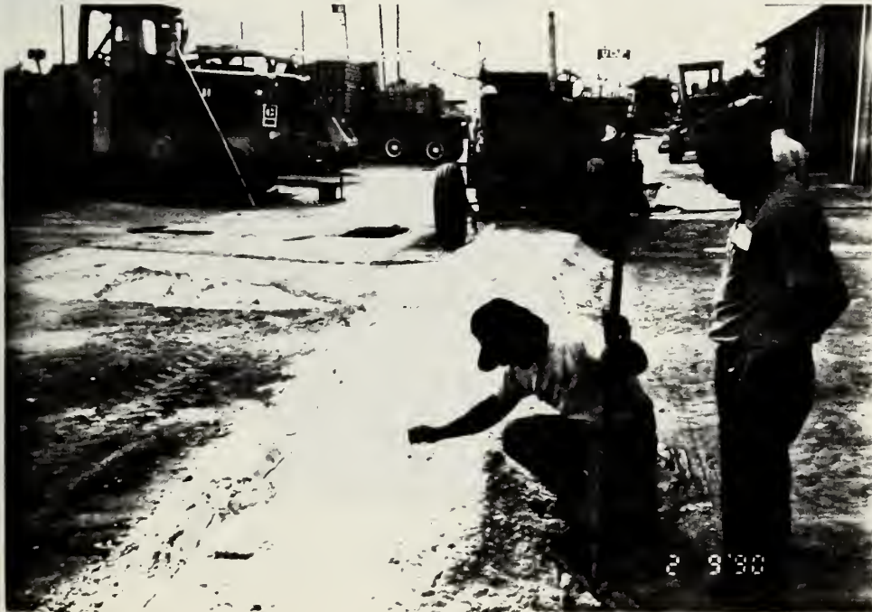
Figure 2.9 Sand Leveling Off and Measuring
